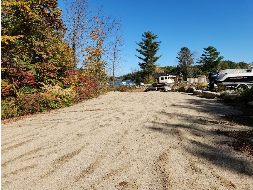
Photo 12: October 2022 - PCB excavation area covered with sand and marker barrier.
